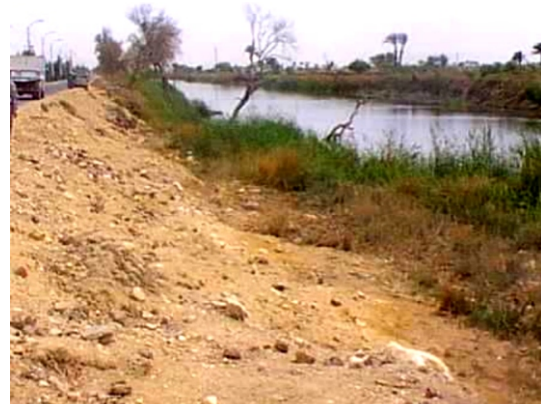
Figure 7 : Slope failure of case 4
