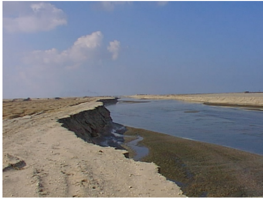
Figure 6 : Slope failure of case 3
