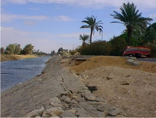
Figure 4 : Slope failure of case 1
