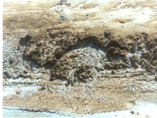
Figure 5 : Salt leaching and slope failure of case 2
