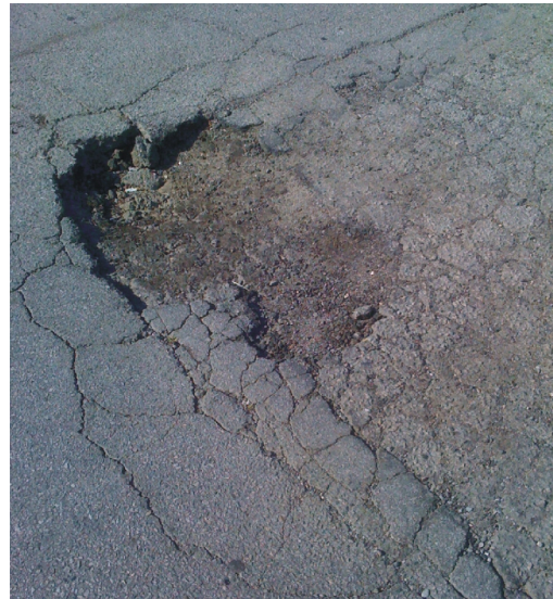
Figure 2 : Stripping in asphalt pavement due to lack of bond b/w asphalt and aggregate
