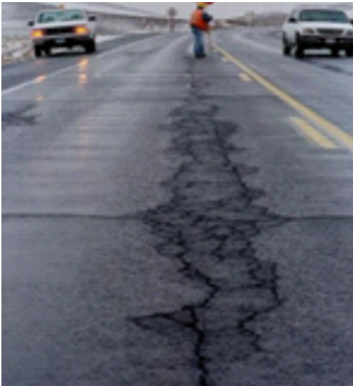
Figure 1 : Fatigue cracking due to stripping in asphalt pavement
